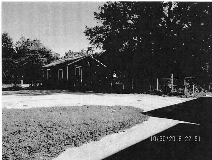
Adjacent residential structure
